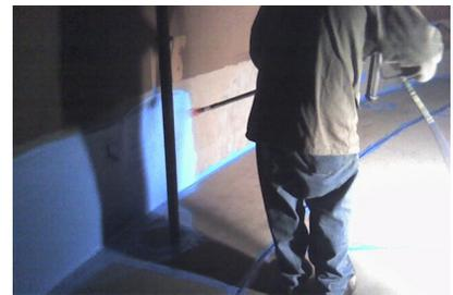
The Tank Armor lining system applied to the interior of an ethanol fuel storage tank at a Massachusetts refinery offers excellent resistance to 100% ethanol over a wide range of temperatures.
