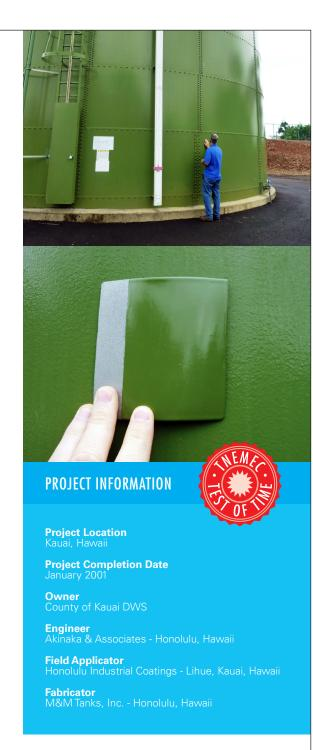
After almost 20 years of exterior weathering in tropical sunlight, hot weather, humidity and frequent rains, the gloss and color of the Series 700 HydroFlon topcoat applied to the Kakela water storage tank in Kauai, Hawaii, remain intact with no noticeable change. Photos shown were taken in 2011.
