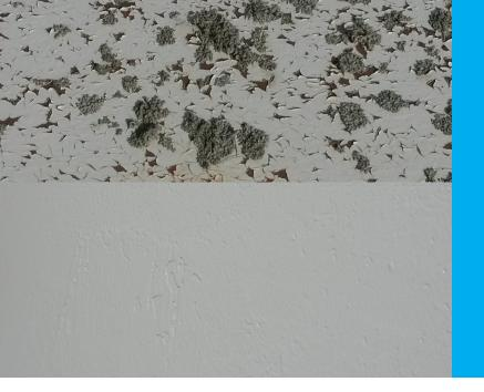
OVERCOAT OPTION Overcoating any existing coating system can result in significant cost savings compared to abrasive blasting and a full repaint, which is often recommended for API-650 tanks.
