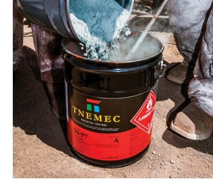
accelerator is available to speed up the curing process, allowing the product to be topcoated "same-day." Additionally, organic zinc-rich primers like Tneme-Zinc do not require a mist coat to prevent out-gassing, allowing for a more efficient application and leaving the topcoats with a consistent and level film.
