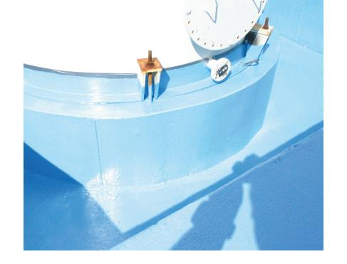
Tank Armor products have been tested in accordance with the MIL-PRF-23236C Edge Retention Test and maintain at least 70% of the film thickness around edges. Coatings that provide good coverage over these edges and protrusions — places where corrosion and coating failures tend to originate — will maintain barrier protection and help prevent costly repairs.
