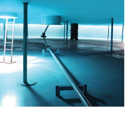
Series 335 Tank Armor has passed DEF testing, tested in accordance with ISO 22241 for its compatibility with AUS 32. Its thick film also showcased excellent performance during steamout testing, mimicking the 20-year cleaning cycle for a pressurized vessel.
