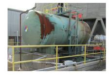
The location and elevated temperature of this sulfuric acid tank caused accelerated corrosion on the steel before being repaired and recoated using Tnemec's innovative thermal insulating coating system, Aerolon.
