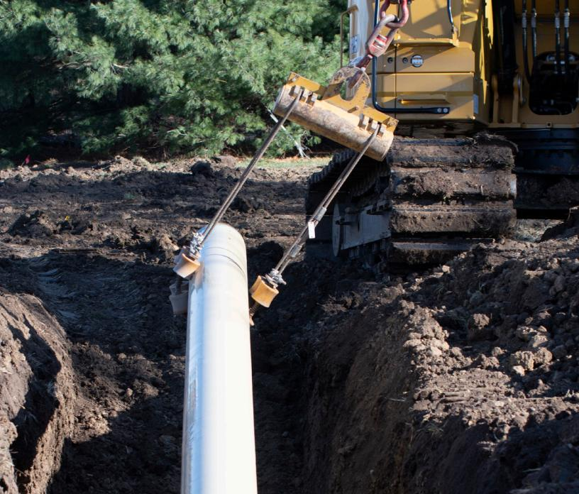
**Above** Series 425 was applied at 40.0 mils DFT on approximately 22,000 lineal feet of pipeline in Schererville, IN. The pipe was then transported to the Kansas City area and pulled through a bore path in a horizontal directional drilling operation.
