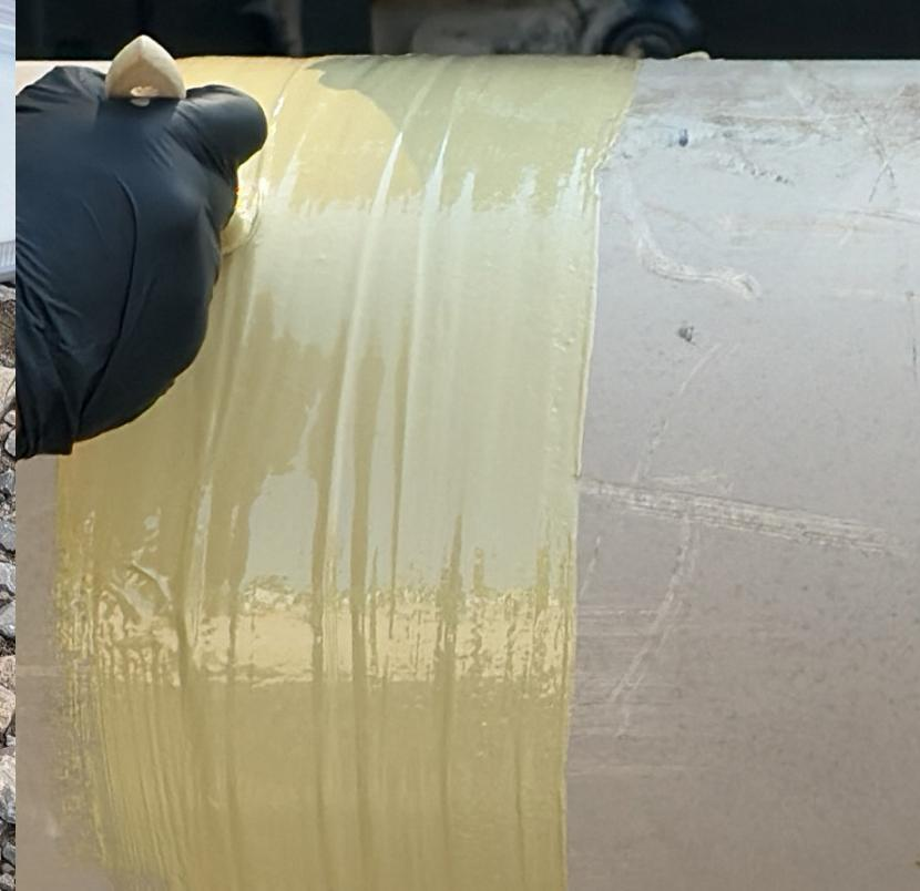
**Above** According to the owner's specification, Series 423 was applied to girth welds on five miles of 12-inch pipe prior to install via horizontal directional drilling in Kansas City, MO. The crew reported excellent field performance and gold-standard support from Tnemec.
