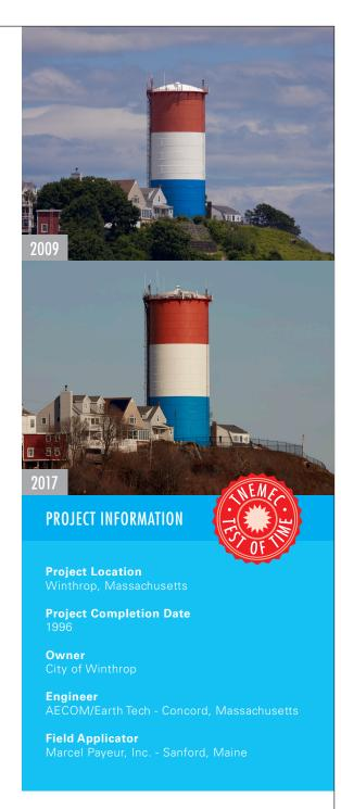
The Tnemec coating system applied in 1996 to the exterior of the standpipe in Winthrop, Massachusetts still looks great after more than 20 years of exposure in a very demanding environment.
