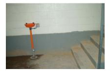
Series 275 Stranlok, a fiberglassreinforced novolac epoxy, protects the concrete at the West Shore Regional Water Treatment Plant from acids, alkalis and other aggressive chemical solutions.
