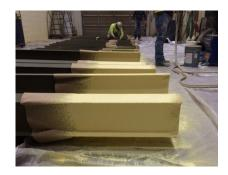
Tnemec's thermal insulating coating, Aerolon, was applied to steel beams for a Pennsylvania student union to mitigate thermal bridging and limit condensation within the building.
