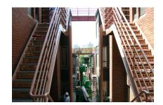
Series 27WB Typoxy was chosen to protect the railings at the University of Georgetown because of its low odor and ease of application over previously painted surfaces.
