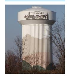
Series 700 HydroFlon, a fluoropolymer polyurethane finish, protects the exterior of the Southeast Highland Elevated Tank in Delaware, Ohio.
