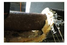
After discovering severe corrosion under insulation in the Omohundro Water Plant, engineers applied the Aerolon coating system from Tnemec to resist future issues involved with CUI.
