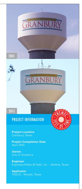
Series 700 HydroFlon was the exterior topcoat of choice for the water tank in Granbury, TX.
