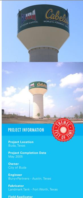
Series 700 HydroFlon, a fluoropolymer polyurethane finish coat, protects the exterior of the Cabela's water tank in Buda, TX, while Series 141 Pota-Pox 80, a high-solids polyamine epoxy, protects the interior.
