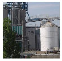
A dry-fall coating system from Tnemec, featuring Series 35 HydroPlate, protects the grain leg and conveyor steel at the ADM facility in Cedar Rapids, Iowa.
