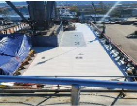
(Top) The Coastal Trader deck was primed with Series N69F and taped off in preparation for the application of the underlayment.
