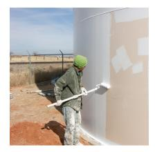
A fast-curing product was needed for the Alabama Avenue ground storage tank, which is why Series 740 UVX was chosen as the exterior topcoat.
