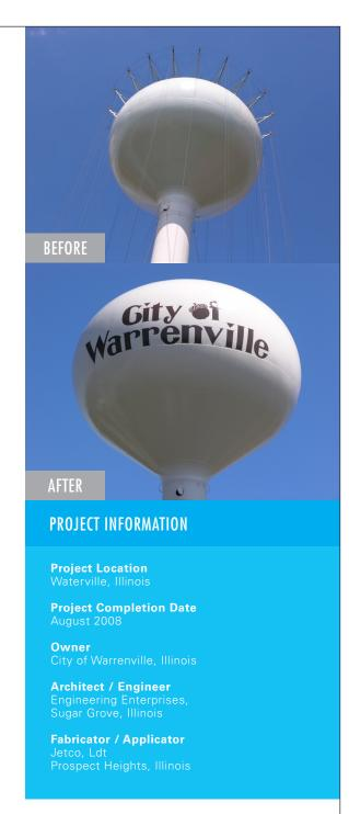
Tnemec's HydroFlon was chosen to protect the exterior of the Warrenville, IL waterspheroid because it offers superior long-term color and gloss retention.
