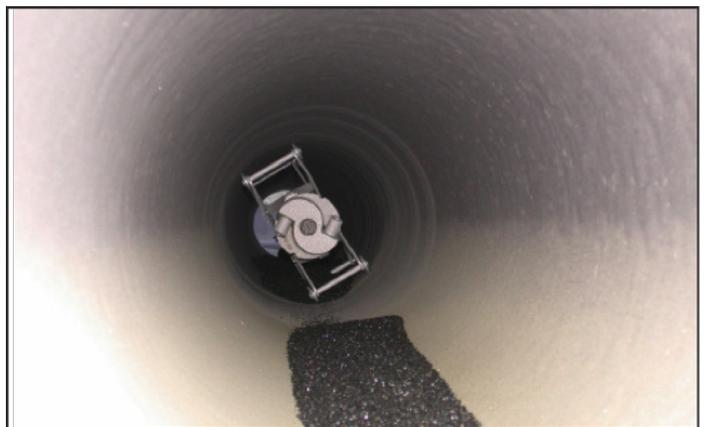
The compressed air used for blasting shall be free of water and oil. Adequate moisture traps and separators should be used to ensure elimination of all contaminants. Cleanliness of the air supply should be checked daily by operating the line without abrasive media through blotter paper for 30 seconds (reference
