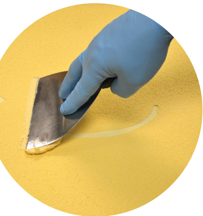
1. APPLY AEROLON TO DAMAGED AREA.
