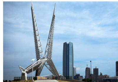
Aside from the stainless steel feathers, all steel on this pedestrian bridge in Oklahoma City is protected by a fluoropolymer coating system from Tnemec. Photos courtesy of David Cobb.
