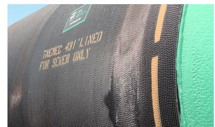
The City of Hobbs Effluent Booster Station used approx. 560 gallons of Series 431 Perma-Shield PL to protect wastewater pipes and fittings.
