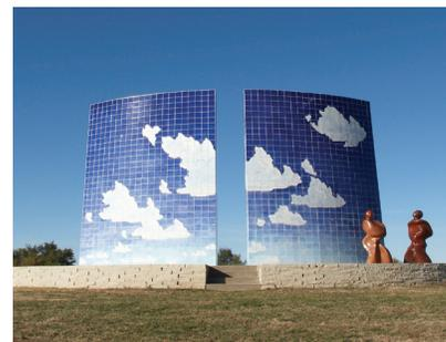
The Newton, Kansas water tank was chosen as Tnemec Company's 2010 Tank of the Year for its impressive exterior artwork that mimics a popular sculpture, also in Newton (above photo), and use of a high-performance coating system featuring a fluoropolymer topcoat for extended protection against the elements.
