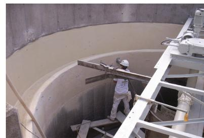
A Perma-Shield lining system was used at the WWTP in Gloucester, MA to protect the concrete from H<sub>2</sub>S gas permeation.
