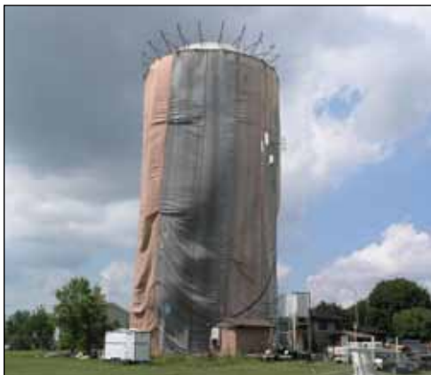
Tnemec's HydroFlon was chosen to protect the exterior of the Warrenville, IL waterspheroid because it offers superior long-term color and gloss retention.
