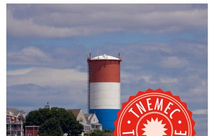
The Tnemec coating system applied in 1996 to the exterior of the standpipe in Winthrop, Mass. still looks great after more than 13 years of exposure in a very demanding environment.
