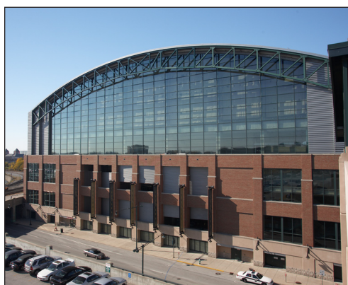
Tnemec coatings protect the structural steel at Conseco Fieldhouse in downtown Indianapolis, home to the Indiana Pacers.
