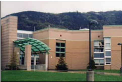
Series 156 Enviro-Crete provides excellent protection for the exterior of the Ecker Hill Middle School in Park City, UT.
