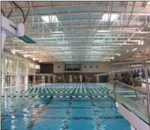
After Hurricane Ivan caused damage at the University of West Florida in Pensacola, Tnemec coatings were chosen to protect the exterior and interior of the rebuilt natatorium.
