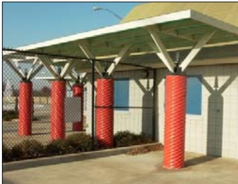
Tnemec and Chemprobe coatings protect the building and entryway at the Earlywine Family Aquatic Center in Oklahoma City, OK.
