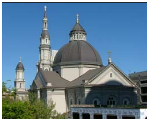
Before, during and after photos of the latest renovation of the Cathedral of the Blessed Sacrament in Sacramento, CA, which features Series 156 Enviro-Crete, a modified waterborne acrylate.
