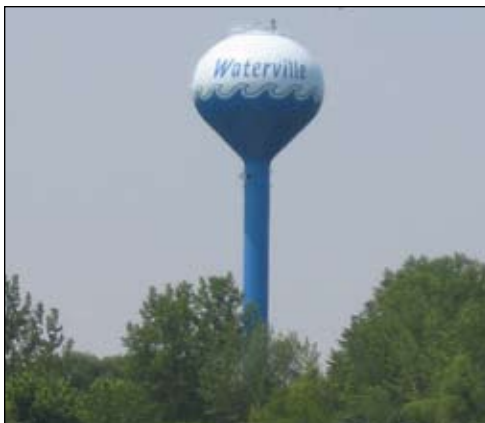
Series 700 HydroFlon, a fluoropolymer polyurethane finish, protects the exterior of the single pedestal water tank in Waterville, MN.
