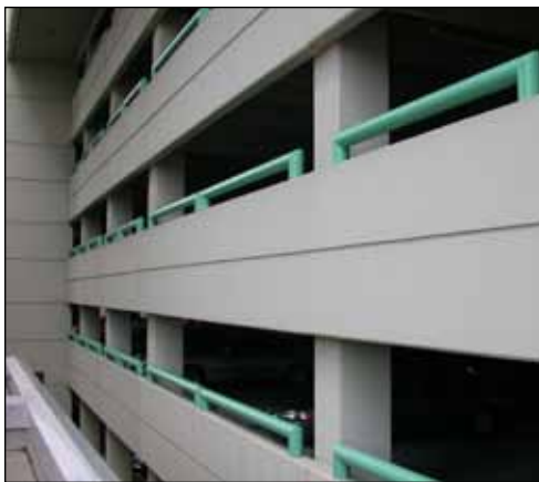
Series 157 Enviro-Crete, a flexible, breathable coating with excellent elastomeric properties, was chosen to protect the RSA Parking Garage in Montgomery, AL.
