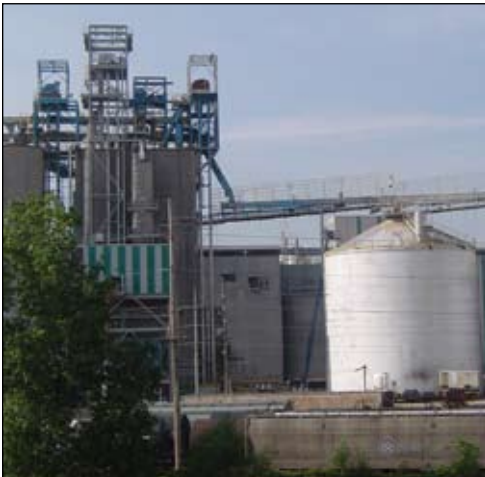
A dry-fall coating system from Tnemec, featuring Series 35 HydroPlate, protects the grain leg and conveyor steel at the ADM facility in Cedar Rapids, IA.
