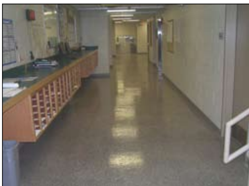
A StrataShield floor coating system including Series 224 Deco-Fleck, Series 284 Deco-Clear and Series 295 Clear CRU protects the concrete floors at the City Hall Maintenance Facility in Eden Prairie, MN.
