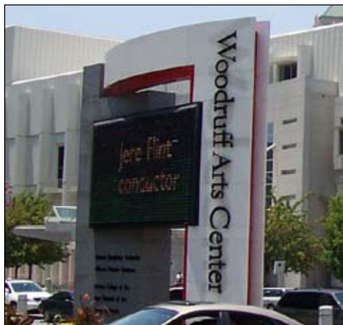
Series 156 Enviro-Crete, a waterborne acrylate, protects the exterior of the Woodruff Arts Center in Atlanta, GA from weathering, alternating freeze/thaw cycles and UV light.
