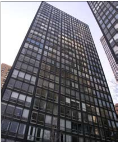
Series 6 Tneme-Cryl, a water-based acrylic emulsion in a charcoal black color, protects the entire exterior steel curtain wall of the towers at 860-880 Lake Shore Drive in Chicago, IL.
