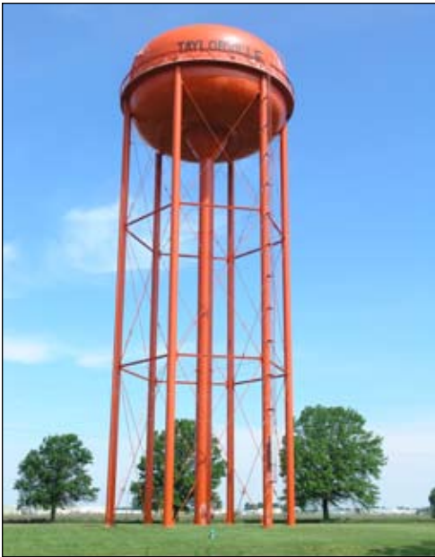
After 15 years of exposure, the Taylorville water tank is still as shiny and orange as the day it was coated!
