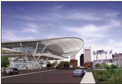
The 12,000 tons of structural steel that support Boston's new one million square foot, $800 million convention center was primed with Tnemec Coating Systems.
