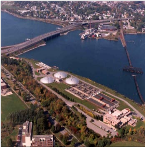
Tnemec coatings protect 42,000 sq.ft. of concrete at the East End Wastewater Treatment Facility in Portland, ME.
