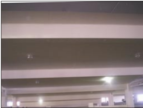
The Employee Parking Garage at the Bellagio Resort in Las Vegas is protected with nearly 34,000 gallons of Series 180 W.B. Tneme-Crete.
