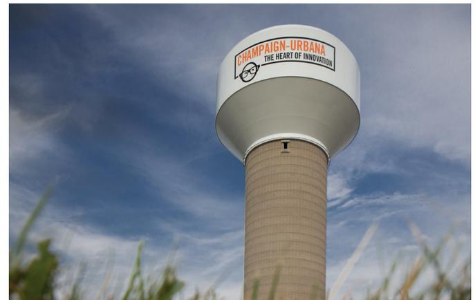
cylindrical shaft support structure. During the summer, when temperatures are elevated, condensation can cause mold and mildew growth, accelerated corrosion and moisture damage to electrical systems and property stored inside the pedestal's base cone.
