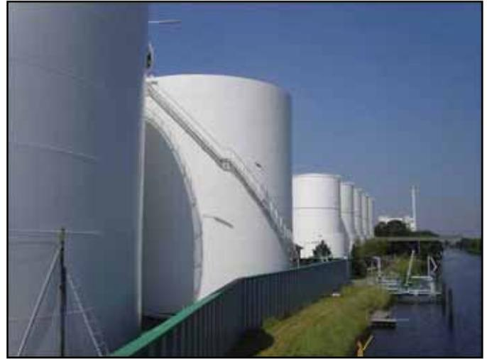
Other low-VOC finish coating options used to enhance color and gloss retention on tank exteriors include Series 1028 or Series 1029 Enduratone, a High Dispersion Pure (HDP) acrylic polymer; Series 740 or Series 750 UVX, a 74 percent solids advanced technology hybrid polyurethane; and a next generation version of Series 700 HydroFlon, a fluoropolymer polyurethane.
