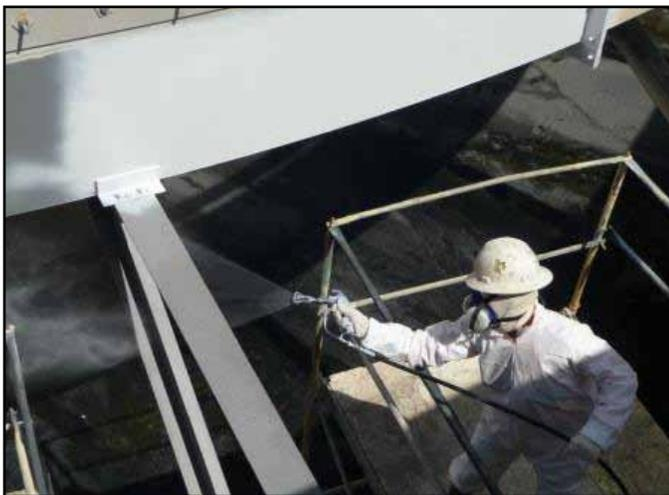
Series 406 Elasto-Shield is a fast-setting, 100 percent solids aromatic polyurethane hybrid lining recommended for immersion service in water and wastewater treatment. Series 406 is also certified by NSF International in accordance with ANSI/NSF Std. 61 for use on the interior of potable water storage tanks and reservoirs of 50,000-gallons capacity or greater and pipes 35 inches in diameter or greater.
